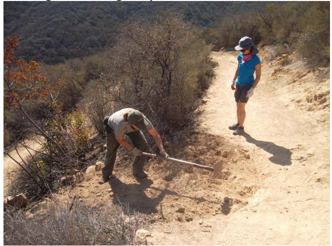
Adding a drainage dip
